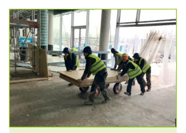
Many manual transport trolleys are available in the market, they are cheap purchasing, but expensive to operate, as a lot of workforce is required to transport the trolley with a load.
